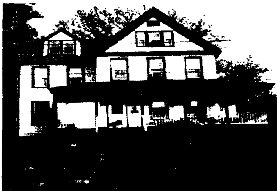
1897 Bradshaw house in Hyattsville, Maryland
